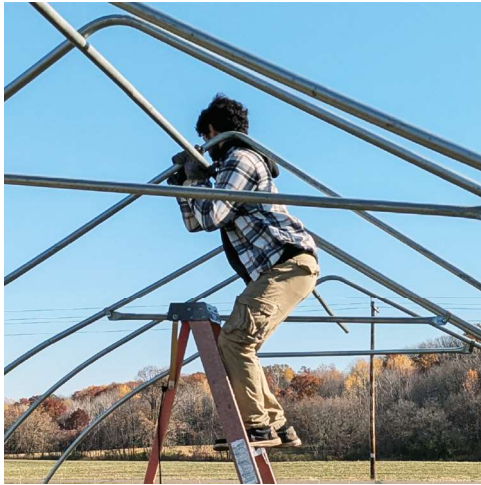
Photo: Elvis up the ladder
