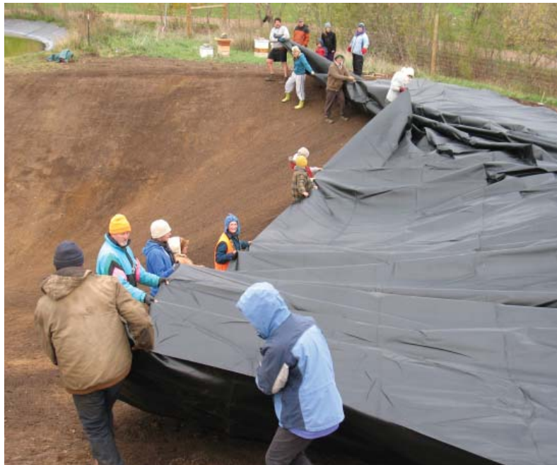
Photo: everyone puts the pond liner in
