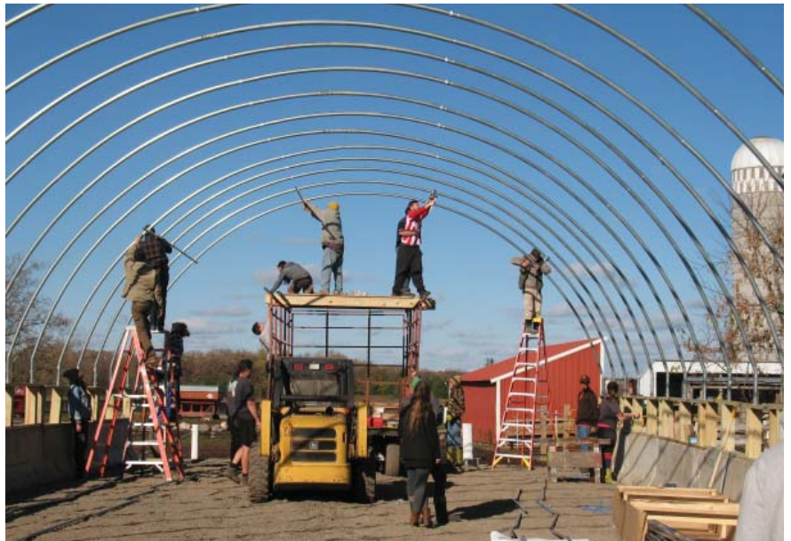
The Mootel going up
