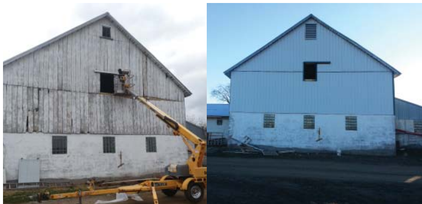
Before and after fixing and siding the north end of the barn
